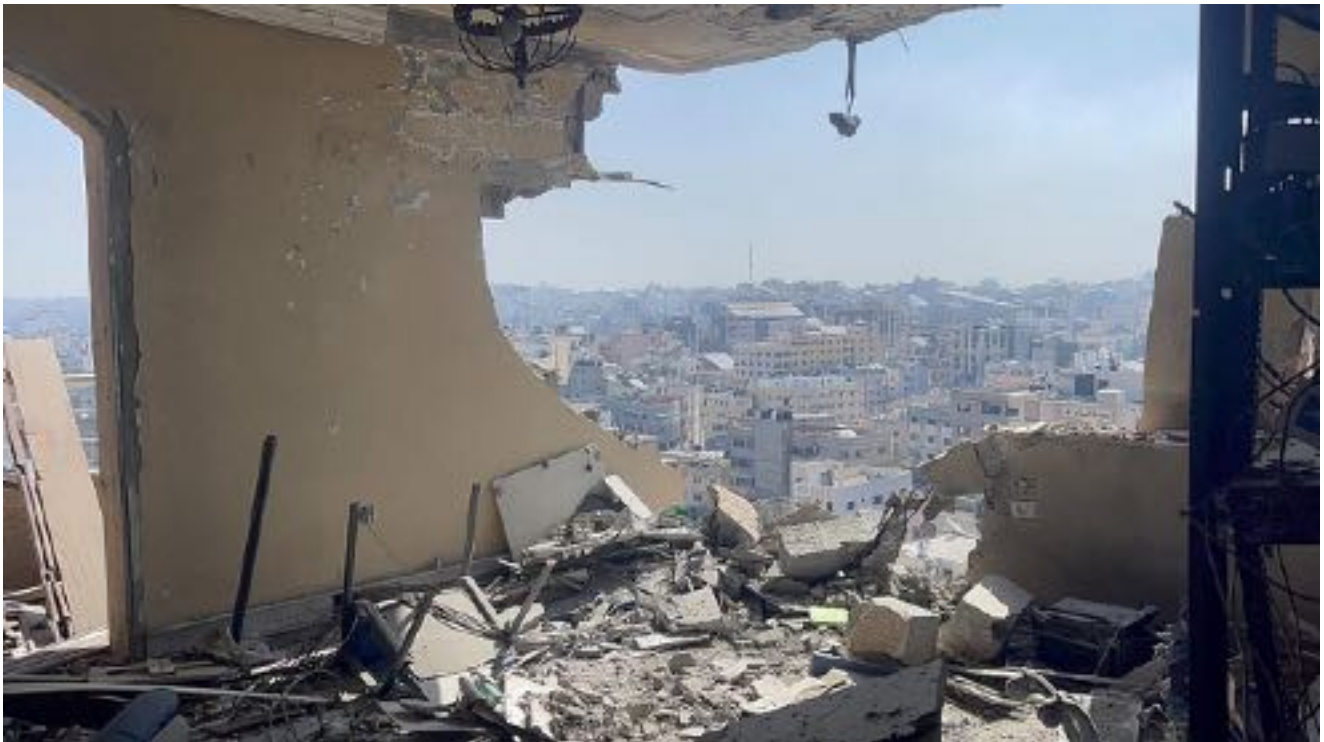
AFP’s server room located on the 11th floor of the Hajji Tower, which was partially destroyed by an Israeli strike on November 2, 2023. (AFP)
